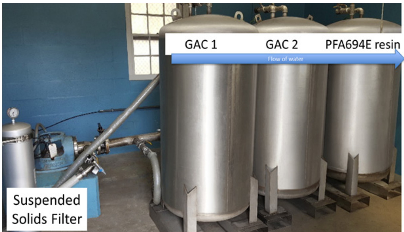
Figure 2. Well 10 Treatment System – Photo courtesy Altair Equipment and Horsham Water & Sewer Authority
