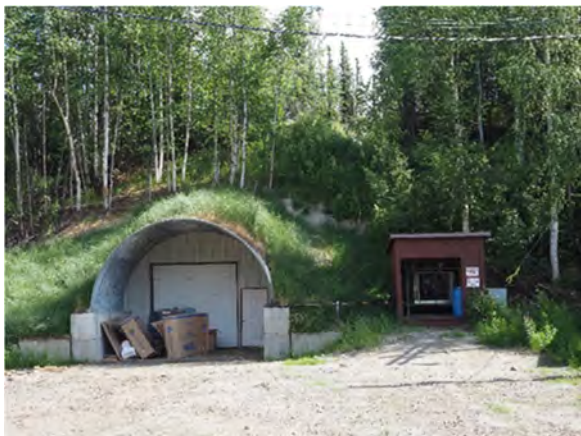
Figure 13. Entrance to the CRREL Permafrost Research Tunnel.
